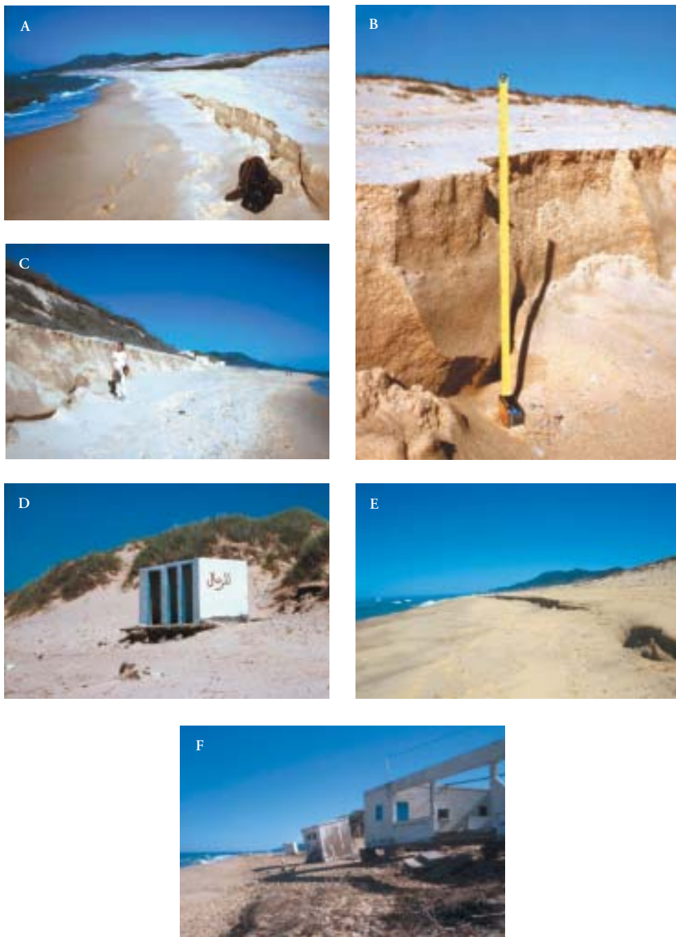
FIG. 2.3.4 (A-F) Degradation of dunes observed at Zouara throughout the study period (1999-2001). (A) Evidence of beach-face erosion (1999). (B) Detail (1999). (C) Significant sediment loss over a span of ten months (2000). (D) Permanent structures as baseline for measuring erosion (2000). (E, F) Accelerated erosion as a result of the disruption of aeolian processes; note scraping of the beach surface (E) and collapse of permanent structures (F) (2001)
